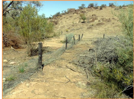
Above – Repairs to fencing
