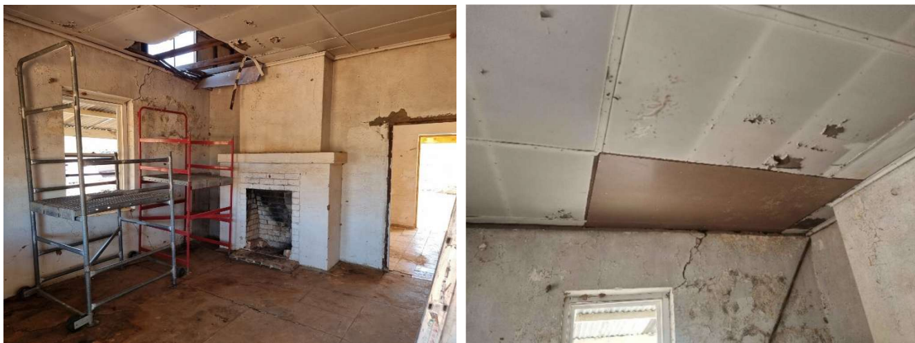
Above: The collapsed ceiling in the “dining room” is now repaired.
