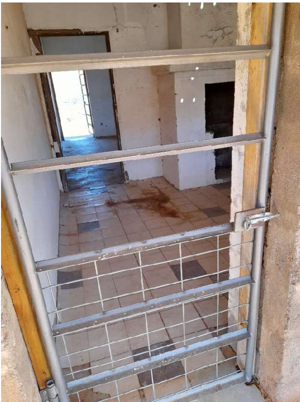
The steel grate acting as an external “door” to the kitchen with anti-kangaroo mesh
