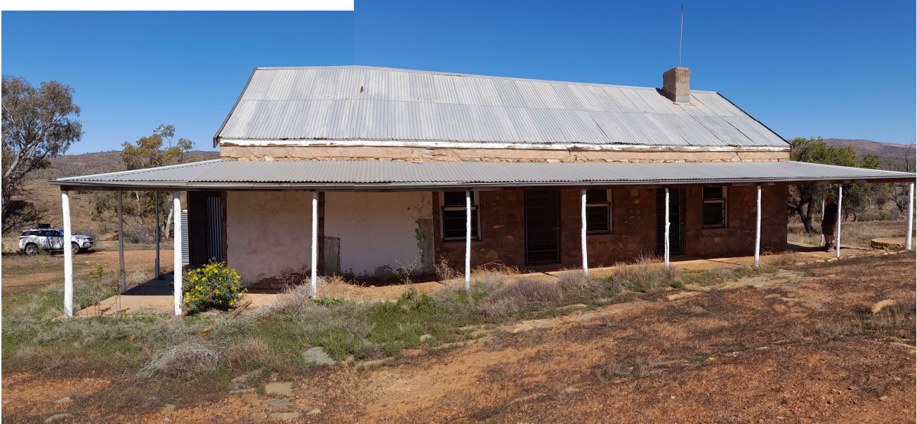
Composite image of the northern façade. A bathroom has been removed from the white-walled area at left. And a laundry room has been removed from under the veranda at right.
